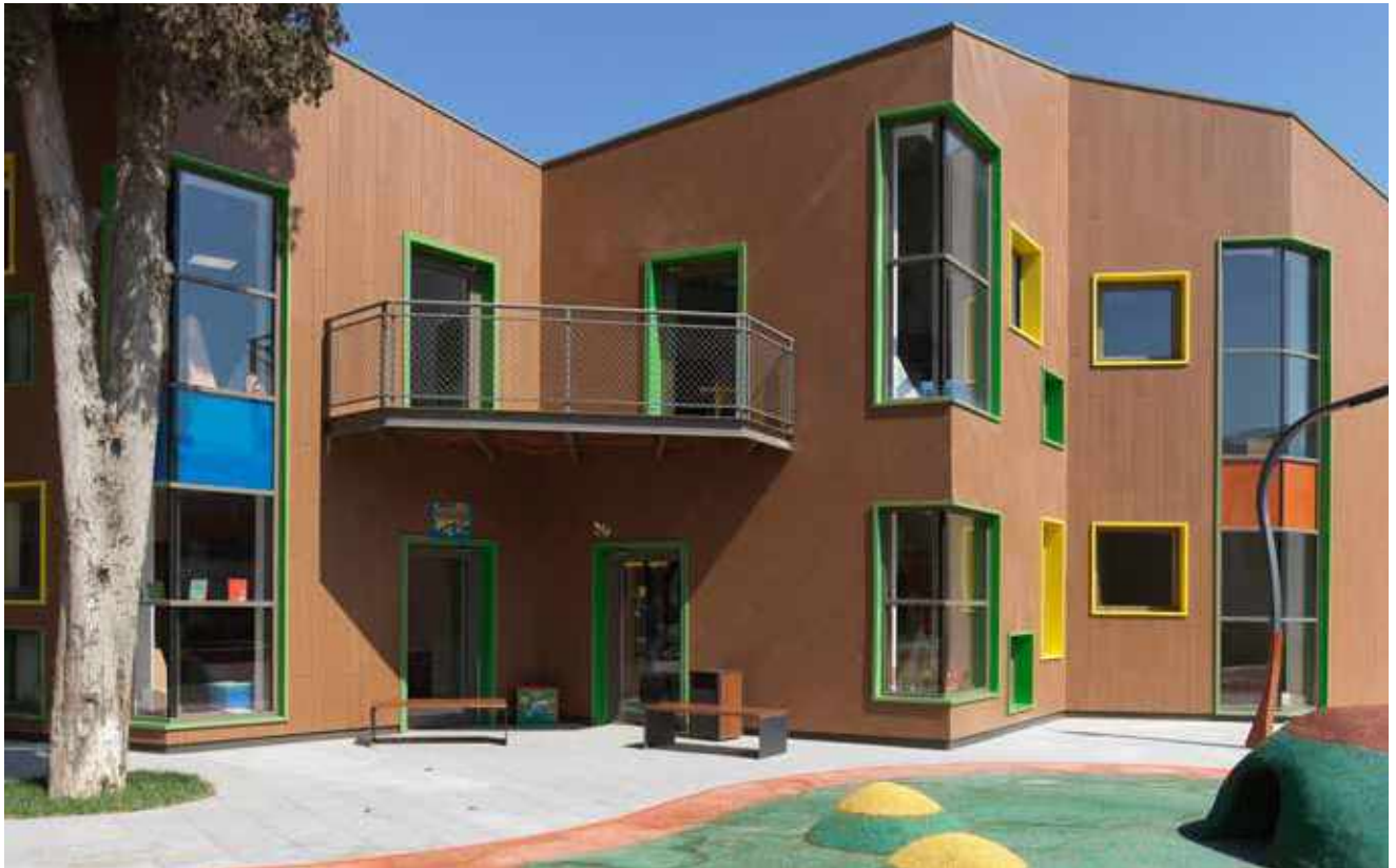
MTK International School in the name of Heydar Aliyev Photography : Cemal Emden
